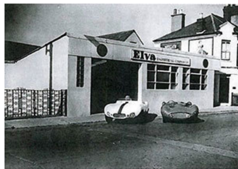
The Elva Engineering ex. London Road Garage showing the roofed over frontage which added to the available workshop space. (1956)
